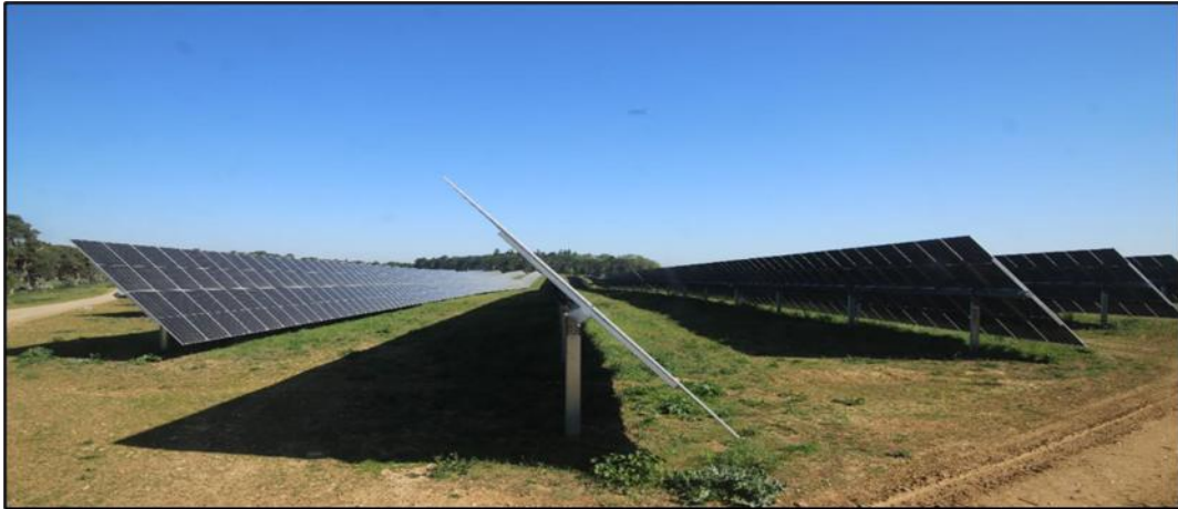
Image 4-2 Typical Tracker Solar PV Panels in a Near Flat Orientation
