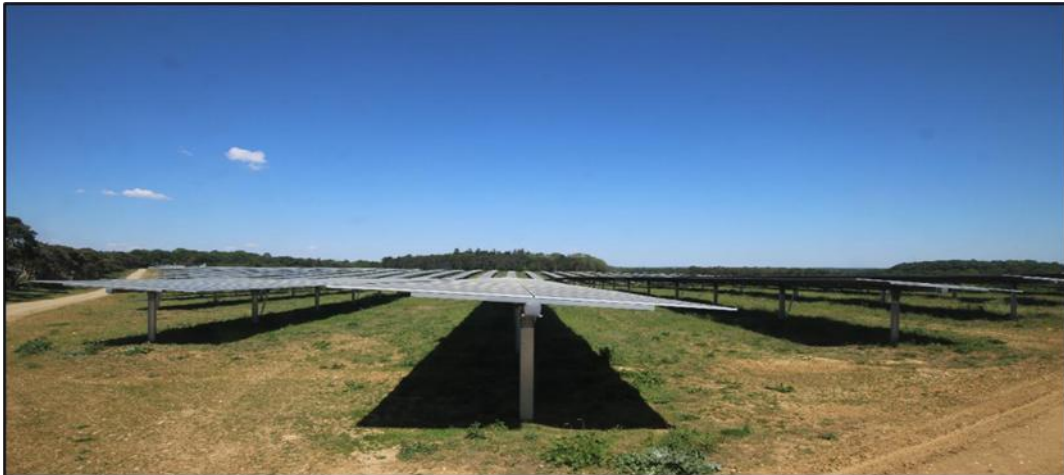
Image 4-2 Typical Tracker Solar PV Panels in a Near Flat Orientation
