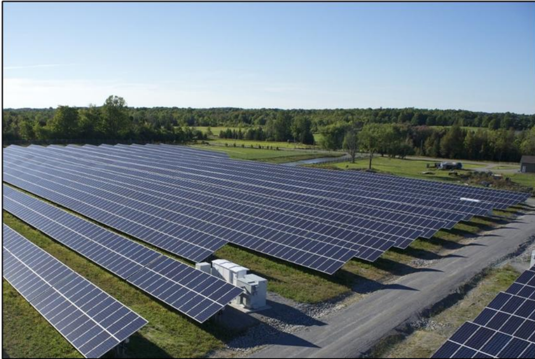
Image 4-3 Typical Fixed South Facing Arrays (with Conversion Unit/Inverter)
